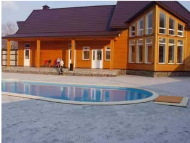
Swimming pool with thermal water
